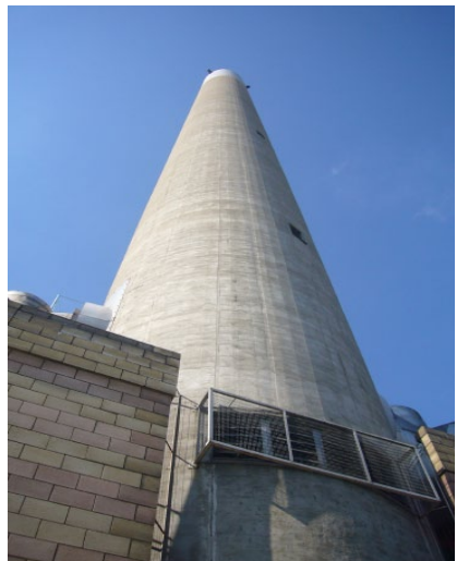
Recycling facility, Bermondsey, London (Picture: Ben Page)
